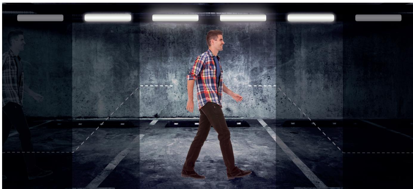
**Corridor function** refers to controlling lighting based on whether motion has been detected.
